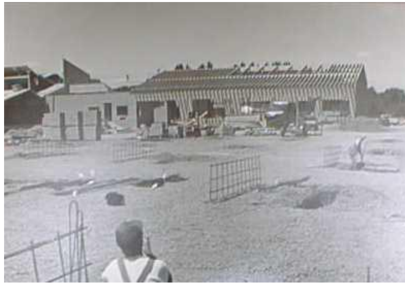
Fig. 12: EPUD under construction
