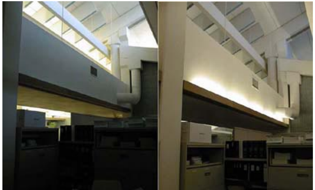
Fig. 46. Illumination measurements were taken with the lights off (left) and lights on (right) on the second floor of the EPUD building.
