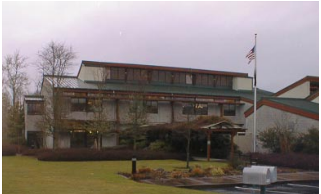
Fig. 4: EPUD Headquarters, south entry
