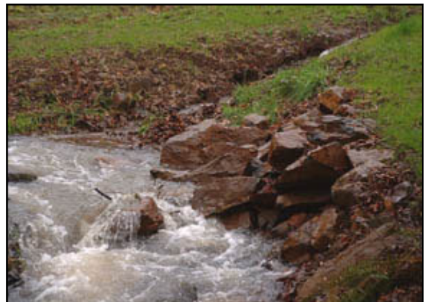
THE MILLERS enjoy the stream that transects their land (left). Rocks were placed on the bend of their stream to reduce streambank erosion (right).
