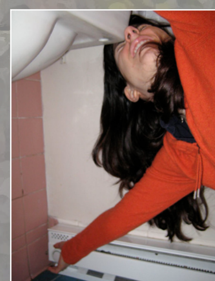
Bathroom heater under sink
