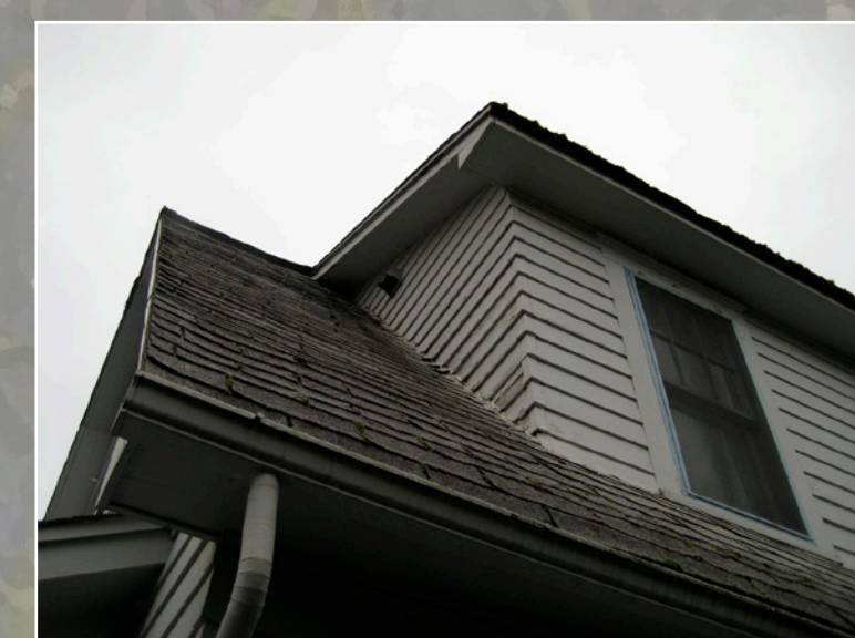
Bathroom window and fan outlet on south side of house
