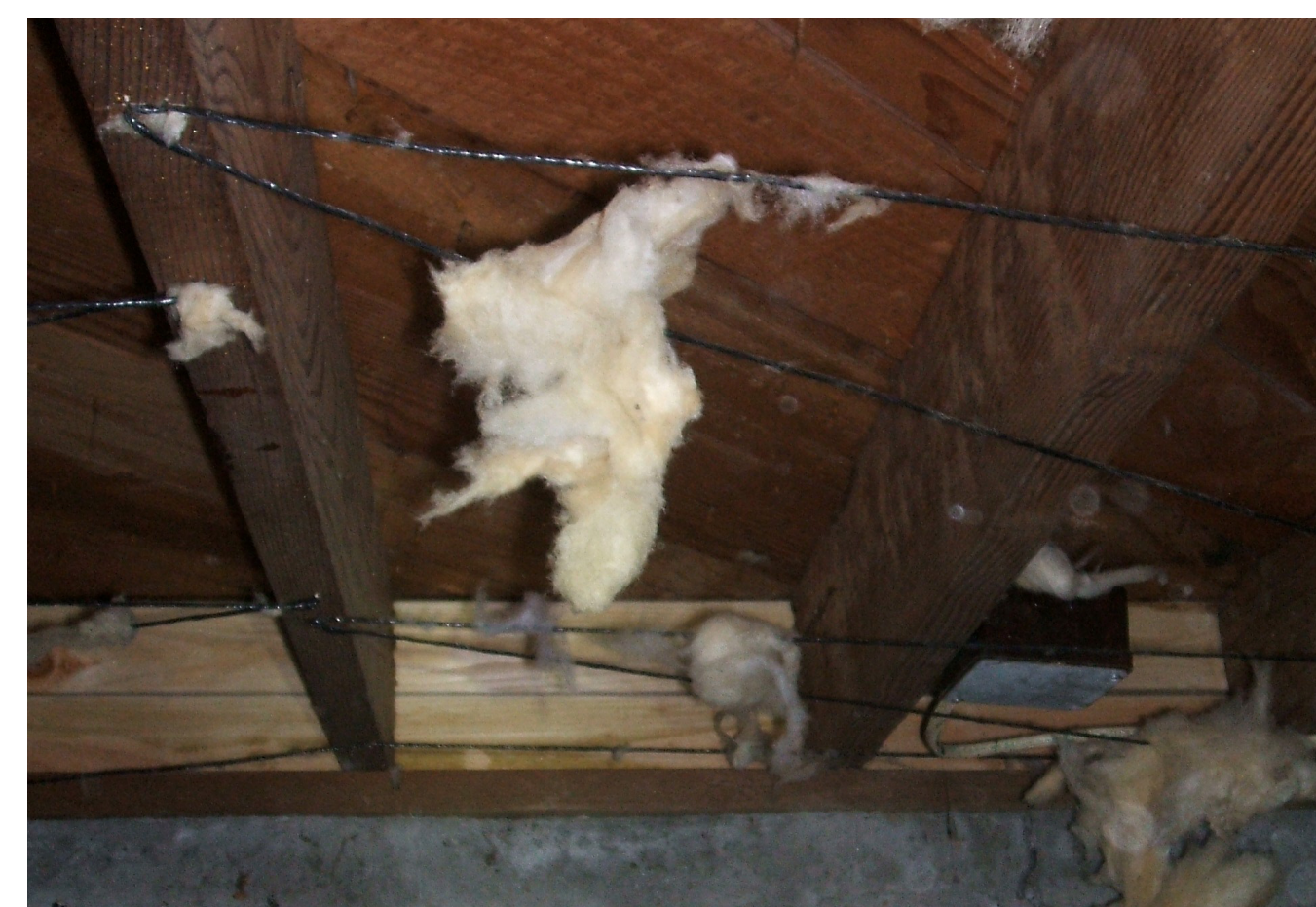
EXISTING CONDITION OF UNDER FLOOR INSULATION
