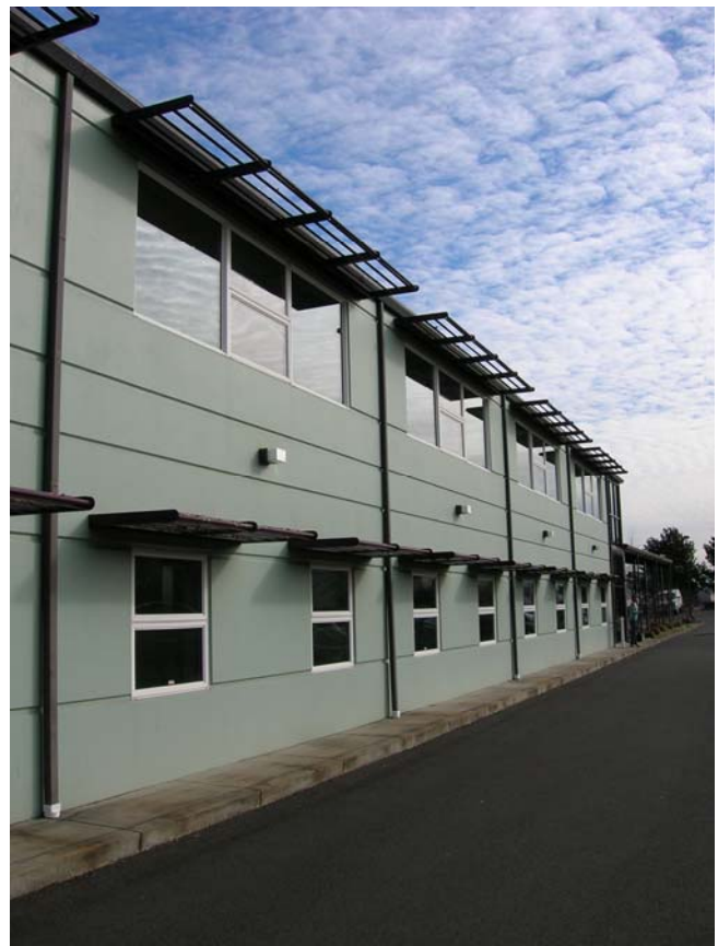
Fig. 1: South façade of the Food For Lane County building.
