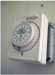
Fig. 3: The bathroom fan timer control
