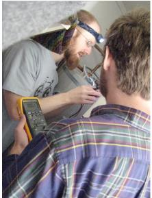
Fig. 4: Removing the bathroom fan timer
