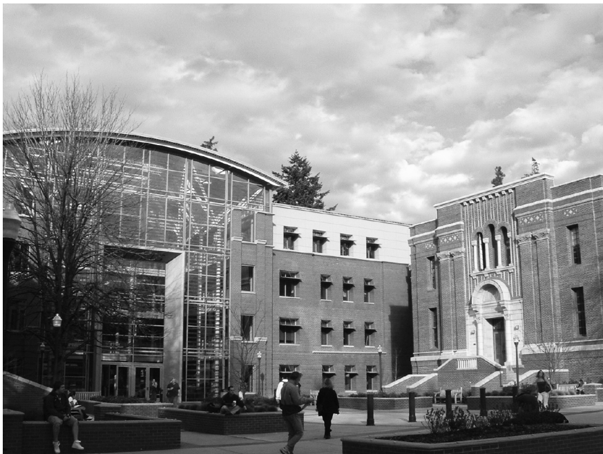
Lillis Business Complex was the first LEED-certified building on campus. It contains a comprehensive mix of sustainable design features.
